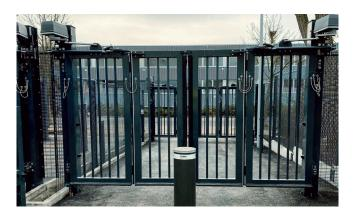
Wherever unauthorized access shall be prevented, but authorized access must be permitted, vehicles are getting locked with 2 gates. The authorized vehicle enters the lock through the first gate. After entering, the first gate closes. Only after the first gate is completely closed, the second gate can be opened. This can happen automatically or via a new verifica-
